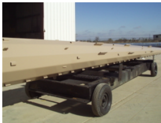
Figure 6. A 100% solids, rigid, aliphatic polyurethane coating used for protection of a communication tower.
